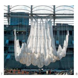
rise high above the structure and which accentuate this location for various events in the imposing skyline of Vancouver (ill. 9). The tiers of seats are covered by a singlelayer membrane consisting of PTFE-coated glass-fibre fabric. The centre of the roof can be opened and closed by means of a twolayer pneumatic cushion structure that is unique in its nature and size.
