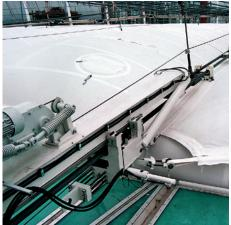
sliding roof in Warsaw, the Canadian structure is in its normal position when closed. The mobile roof, with an oval layout, has dimensions of roughly  $80 \times 100$  m in an extended state. Divided between 36 axes, the individual cushion bays are arranged in radial fashion about a central mast approximately 60 m above the playing field. The mast bears the load of the "garage" or parking space for the roof, into which the membrane can be folded (ill. 12).
